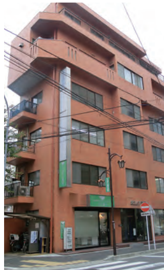
Nagoya Testing Room
